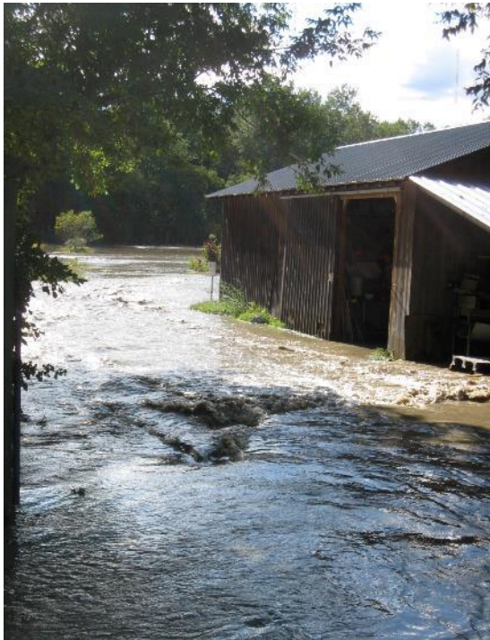
ICF barn during 2011 T.S. Irene flood
